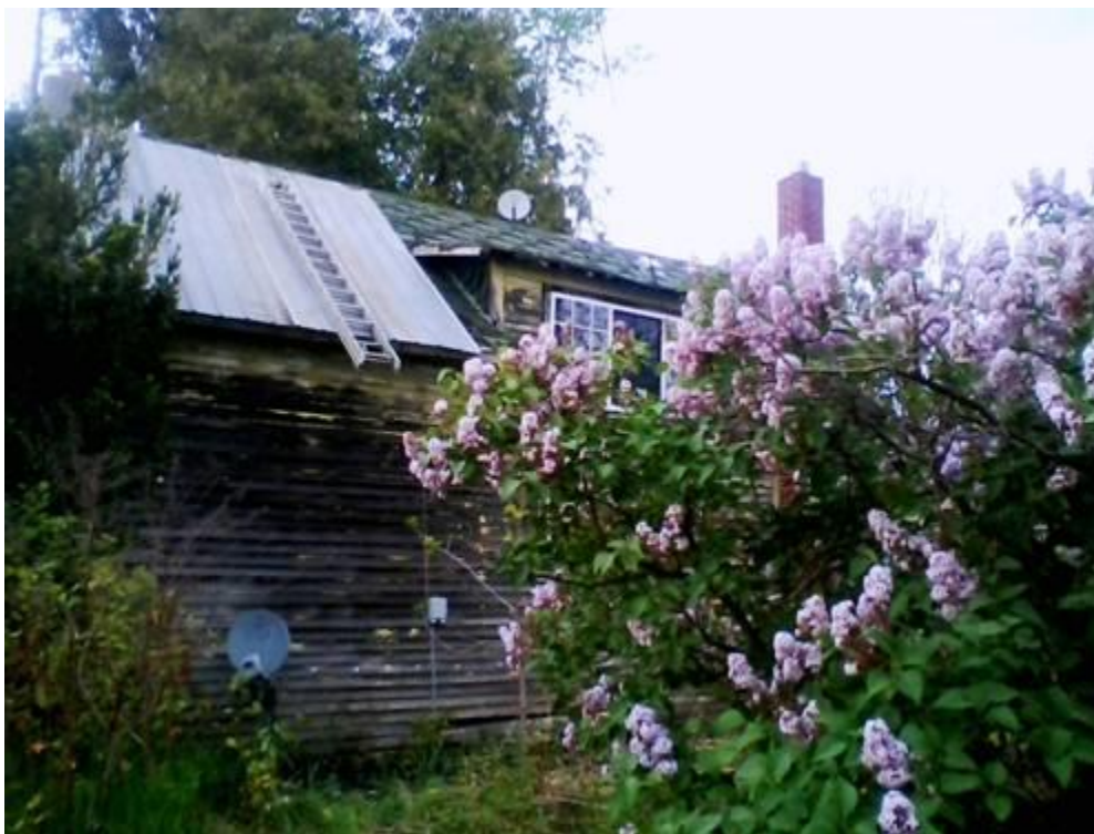
North Street Station
