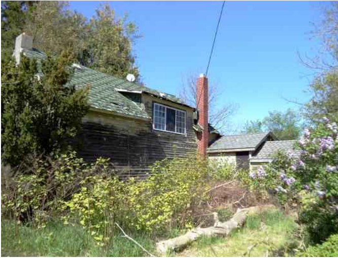
South side of the North Street Station before any restoration was conducted in 2016. The large window was installed and other modifications were made in the mid 1940s to upgrade the structure as a residence.
