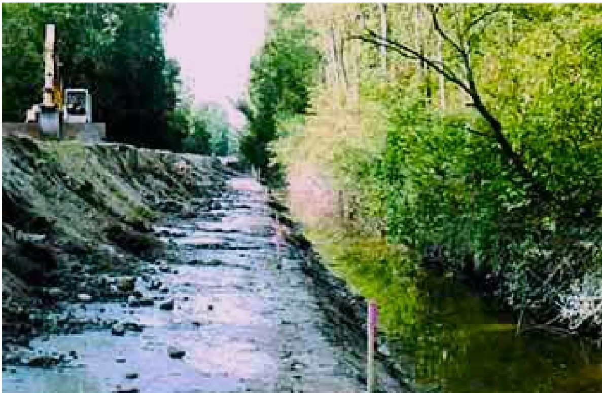
Initial excavation of floodplain shelf. Galbraith Drain at right. Original top-of-bank was about same height as excavator at upper left. Note shallow groundwater seepage from sand (left) across lakeplain clay (middle). Photograph by Bill Collins, 2004 August 24.
