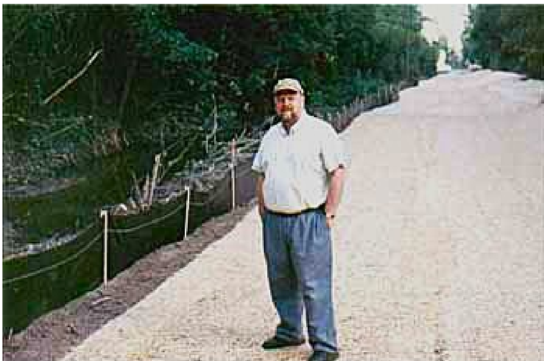
Saint Clair County Drain Commissioner, Fred Fuller, standing on erosion control matting installed on new floodplain. Galbraith Drain is left of black silt fencing.
